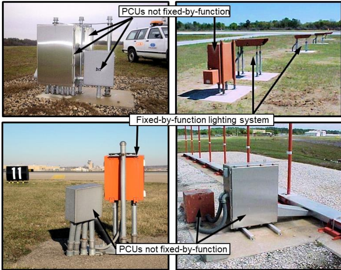
Figure B-4. Equipment Not Fixed-By-Function
